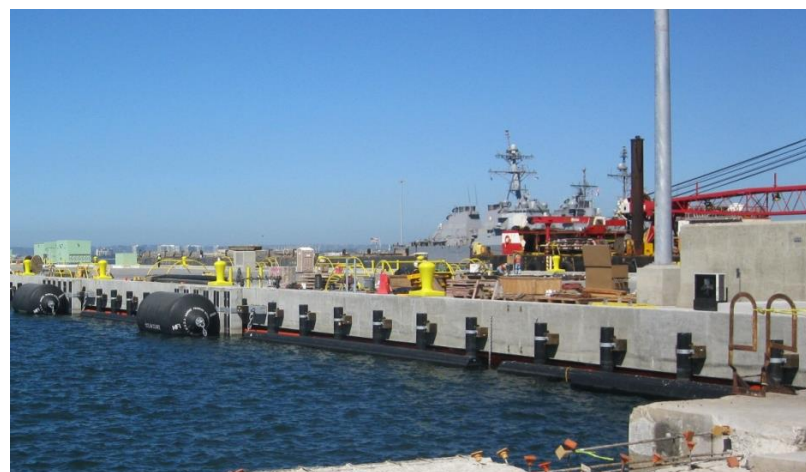
View of Pier 12 with all camels and fendering installed.
