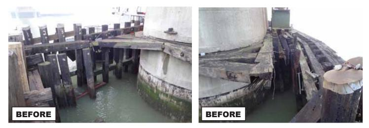
**Challenge:** The Union Pacific Railroad Bridge in Martinez, CA suffered a vessel impact to the Bridge-Pier-Protection System. The Impact broke several of the Wood Piles and Timbers that are part of the original system. Given the strict environmental protection laws in California, repairing with replacement wood piles and or timbers was not an option. An environmentally friendly alternative to creosote treated wood pile/timbers was needed.
