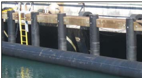
Harbor Technologies HarborPile and HarborCamel installed in Point Loma, CA
