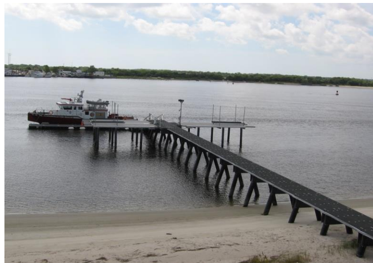
All composite pier designed for hurricane force weather.
