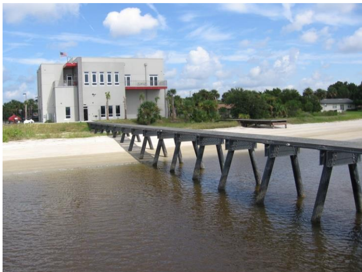
View of Station #40 from pier
