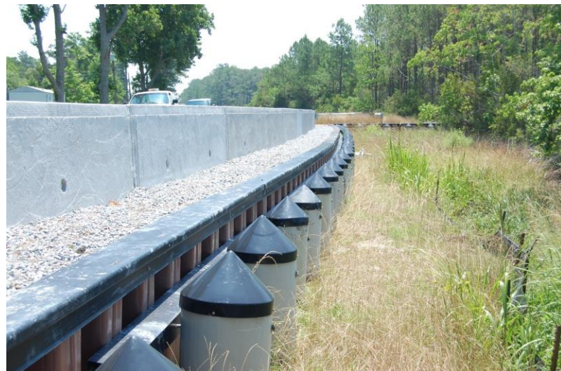
Portion of the 17.7 miles of wall built with HarborPile
