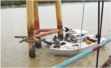
Installation crew in place at low water.
