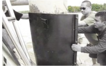
1 min Wrap is positioned.
