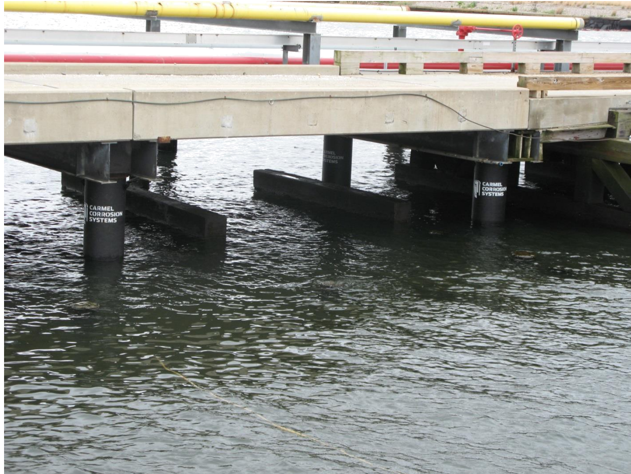
24" vertical piles Photograph taken at high tide.
