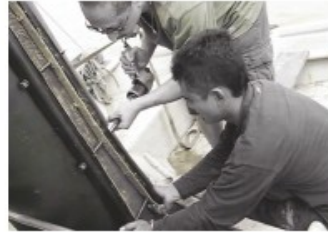
5 min Closing the Flanges.
