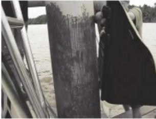
Any marine growth is scraped off pile.
