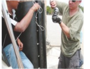
20 min Tension bolts replaced.
