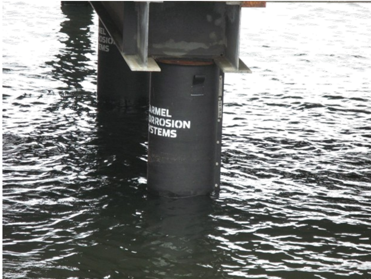
24" vertical piles showing identification plates and vertical lifting lugs.
