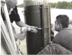
2 min Aligning tension bolts.
